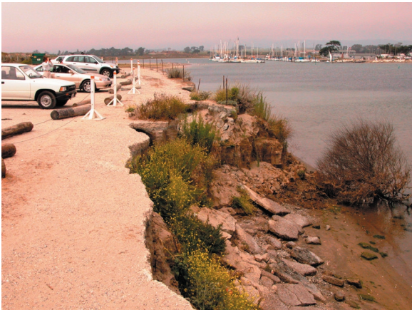
Figure 22. Bank erosion of channel and tidal creeks in Elkhorn Slough causes marsh loss and threatens public access sites.
