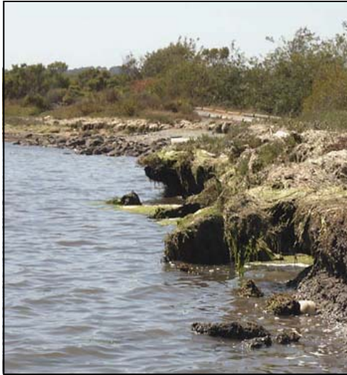
Bank erosion causing marsh loss near Kirby Park
